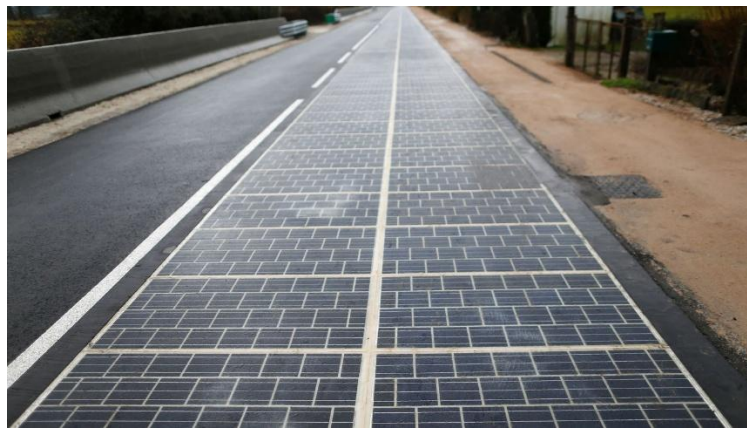
Figure 2.18. Road-attached photovoltaics. (Source: France's Tourouvre-au-Perche)
